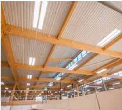
Engineered timber roof and wall cassettes deliver sustainable buildings at a rapid rate, without compromising on quality or efficiency. Our systems offer high levels of prefabrication and integration for accelerated build programmes.
